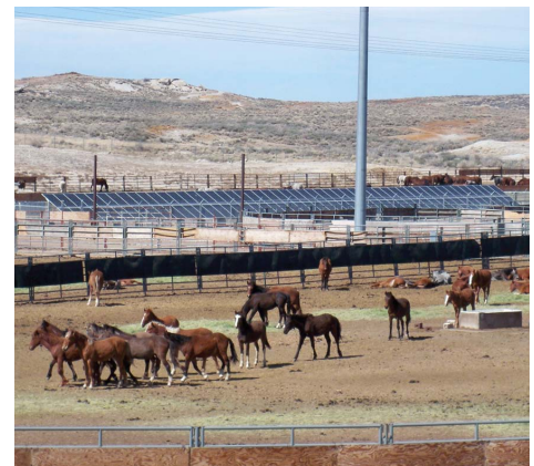
A 25 kW photovoltaic field helps power a horse corral complex in Wyoming.
