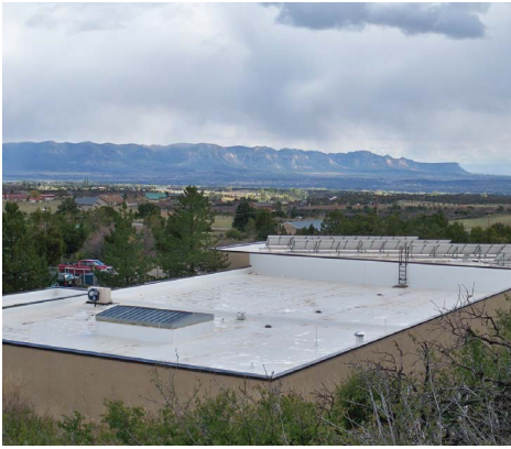
The Anasazi Heritage Center in Colorado includes 38 kilowatts of photovoltaics on the energy-reflecting white roof.
